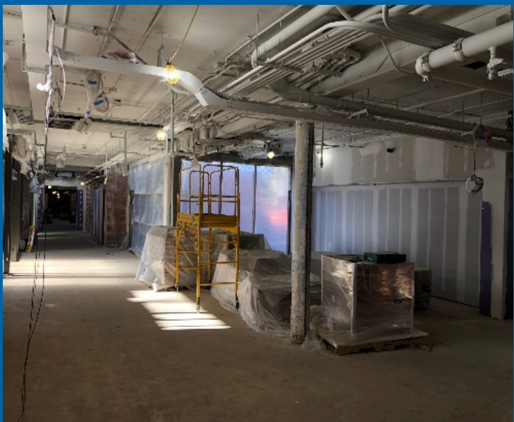
Main Lobby Drywall Finish & Ceiling Paint
