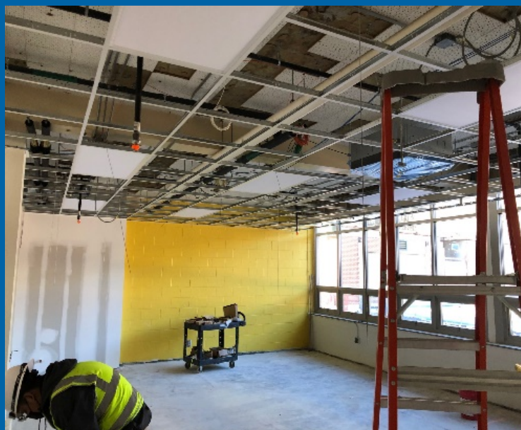
East Wing Ceiling Grid and MEP Trims
